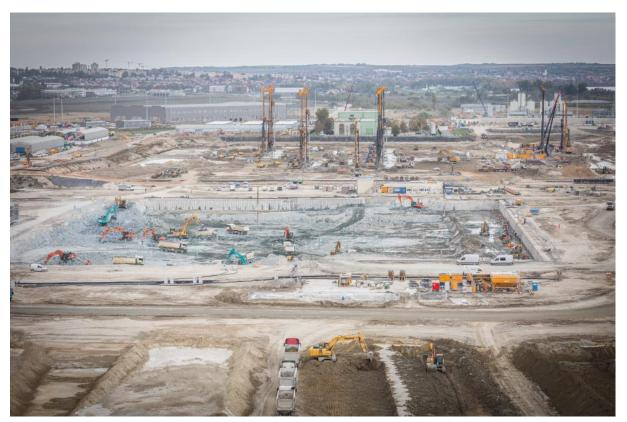
*Construction site of the Paks II. Nuclear Power Plant with excavation to the design level of Unit 5 and soil consolidation work on Unit 6 on October 17, 2024. The photo was taken by Paks II. Ltd.*
